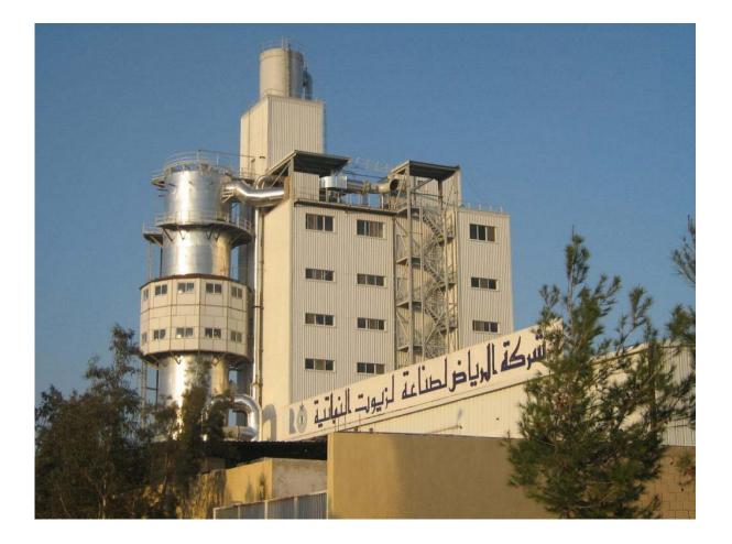
The hot air is conveyed to the lower part of the spraying tower. Two fans, determining the pressure conditions of the air circuit, are installed for regulation of the air-flow passing through the tower. By this circuit the hot air is conveyed via a distribution special rina located at the bottom and from there up to the top of the tower coming into contact countercurrently with the slurry spray falling down from the top.
