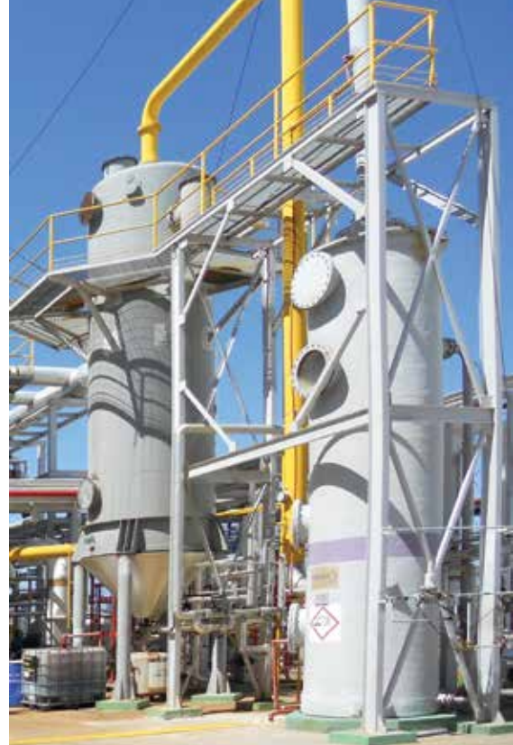
Exhaust Gas Treatment unit based on ESP and SO 2 Scrubber
