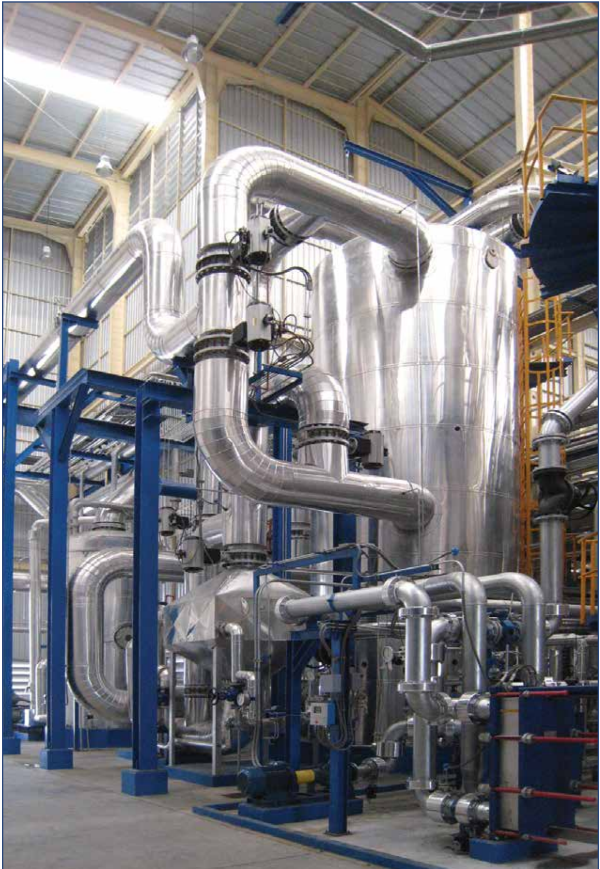
Air Drying and regeneration circuit
